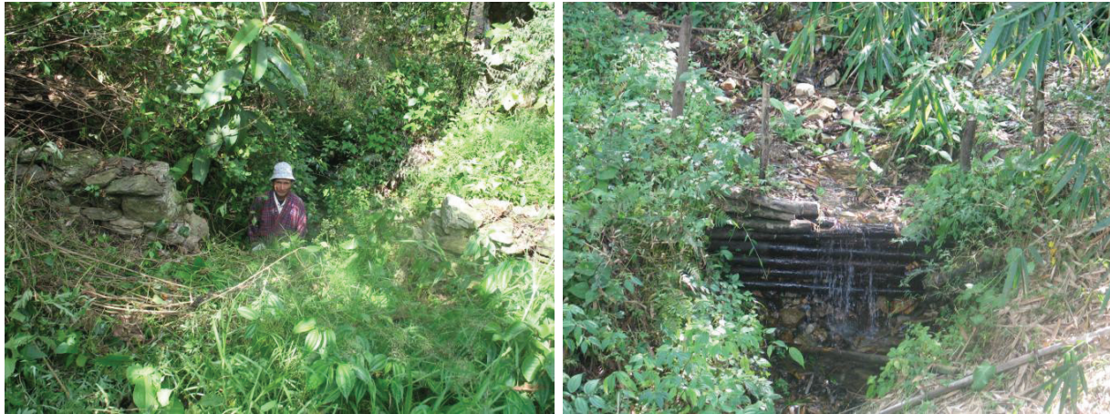
Figure 6.2.5 Gullies stabilized by stone and log check dams.
