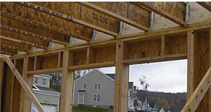
The rim joist for the second-story floor provides adequate structural strength so solid headers are not needed above first-story windows, allowing more room for insulation.
