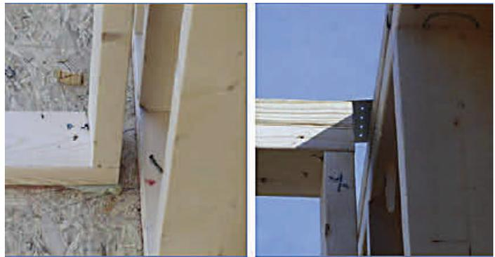
The interior wall framing is anchored to the top plate of the exterior with a flat plate connector.
