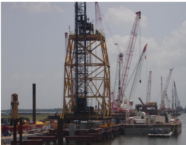
66-inch Concrete Tower Pile Template
