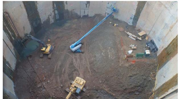
132-foot-diameter dewatering shaft excavation
