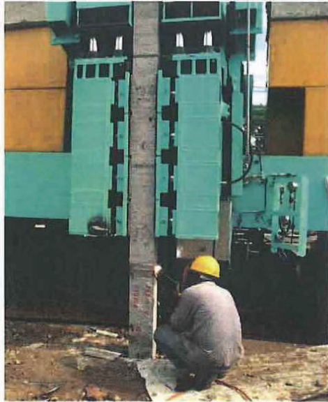
Picture 1: Welding for the joining piles
