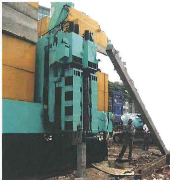
Picture 2: Lifting pile to the gripping position
