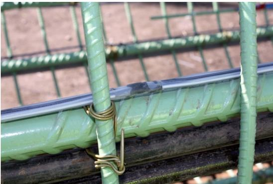
Digital thermal sensor on cable
