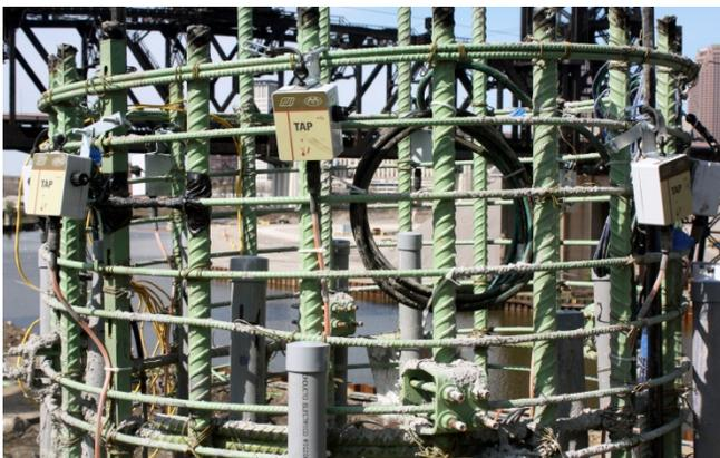
Shaft fitted with THERMAL WIRE cables and data acquisition ports (one per cable)
