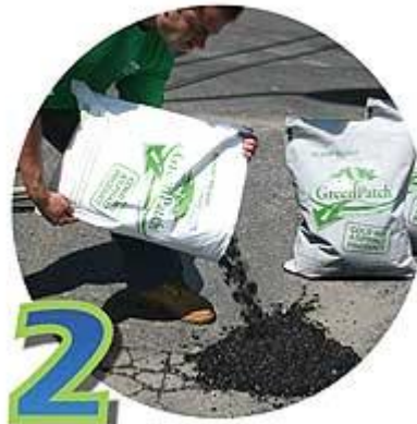
2 Pour GreenPatch directly from the bag into the hole. There are no additional steps or materials needed.
