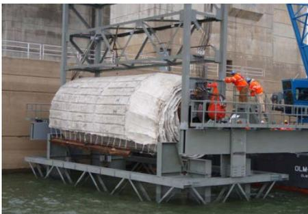
Grout mat being lowered through the guide frame to the river bottom.
