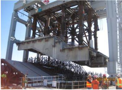
Super Gantry Crane—largest of its kind-- capable of lifting up to 5,300 tons.
