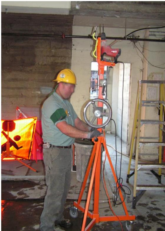
**Figure 3: Overhead drill press in the field**
