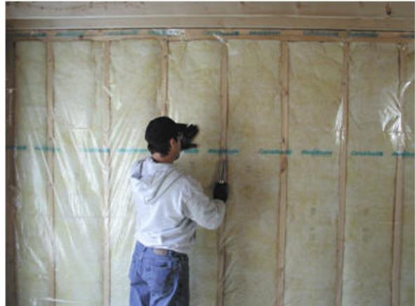
During the heating season when average relative humidities in insulated cavities are typically low, MemBrain works as a vapor retarder.
