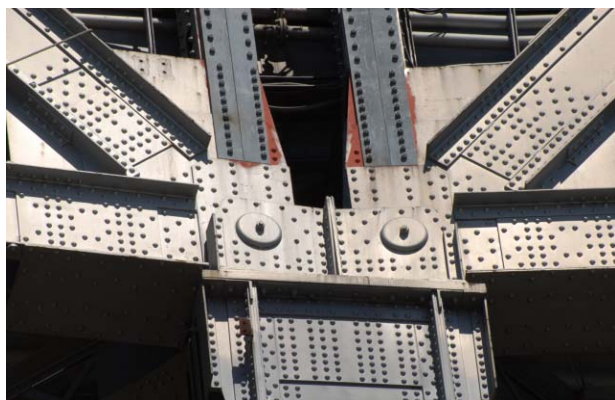
Figure 2: Bolt pattern on the south side of the Bay Bridge
