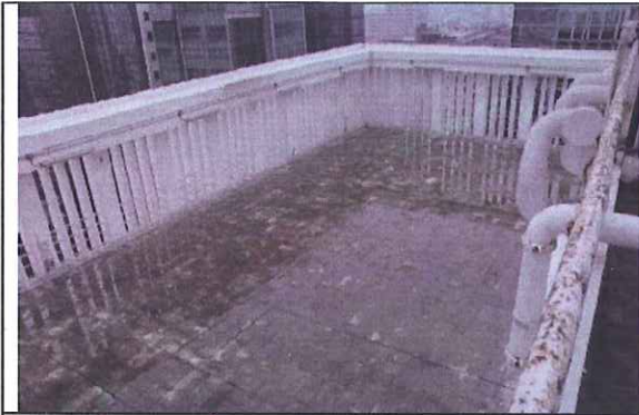
Appearance of roof top before the project
