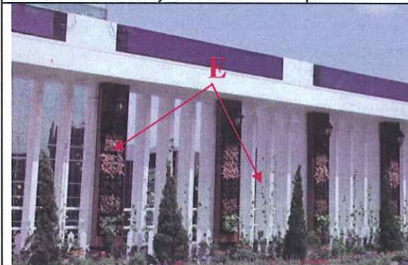
Indicator E: Replaceable box type and wire panel cladding type vertical greening
