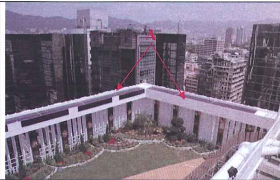
Day view of completed Living Roof Project Indicator A: Renewable Energy – Thin Film Photovoltaic Panel
