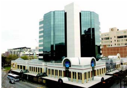
City Centre Office Complex
