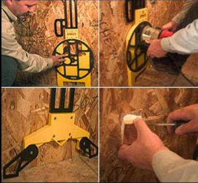
**Cut three different electrical receptacles at three different heights within minutes!**
