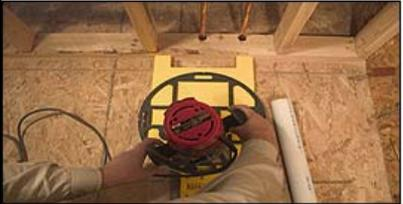
The versatile ZIPROUTE® can also be used to cut water supply and drainage holes.
