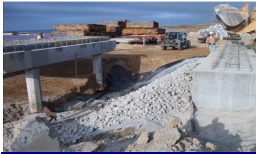
Construction of Pier Foundation
