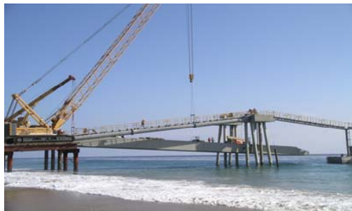
Ramp being hoisted into place
