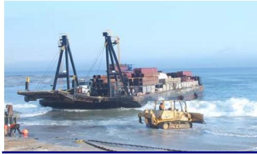
**Original method of beaching barge for Offloads**
