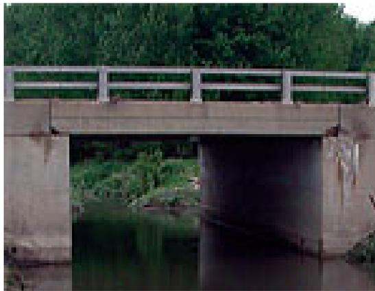
Figure 2. Older bridge showing deterioration due to scour (A typical bridge that would be monitored with the Scourwatch system).
