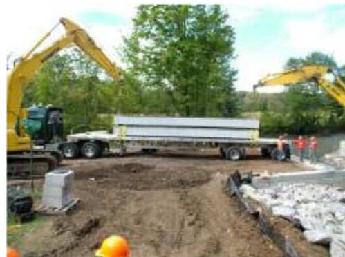
(2) Arrival of Bridge Decks to site
