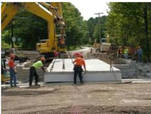
(3) Placement of Decks
