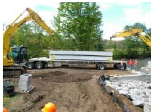
(2) Arrival of Bridge Decks to site
