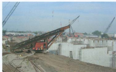
From September 2003 to December 2003, 718 tieback anchors were installed with this tieback machine at Paerdegat Basin CSO Retention Facility, Brooklyn, New York.
