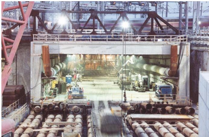
Jacked Tunnel with Passenger Trains Passing Less than 6 ft. above.
