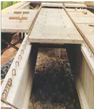
Fig. 3. Conventional SIP Precast Panel System
