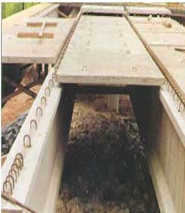
Fig.3. Conventional SIP Precast Panel System
