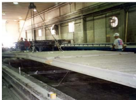
Fig. 7. The NUDECK being lifted from the Prestressing Bed
