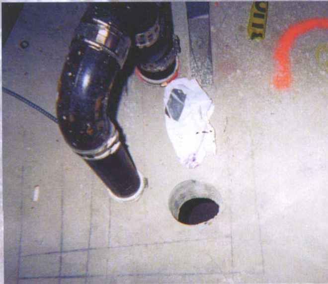
The mechanical contractor is able to drill the hole by staying away from marks which represent cables.
