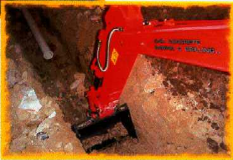
Electric excavator has ability to dig 5' deep.
