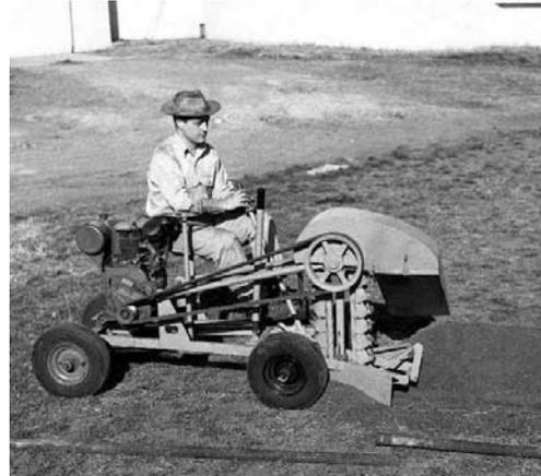
The DWP trencher is used to prepare for the installation of a water line.
