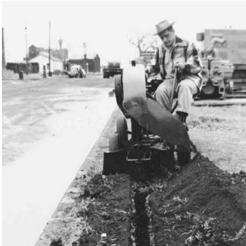
Ed Malzahn digs a 4-inch wide trench with the DWP trencher
