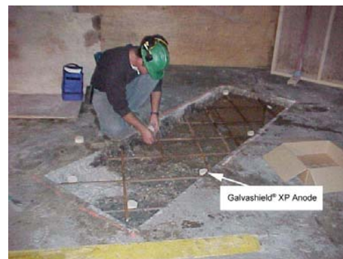
Concrete Patch Repair – Anodes tied around perimeter of repair
