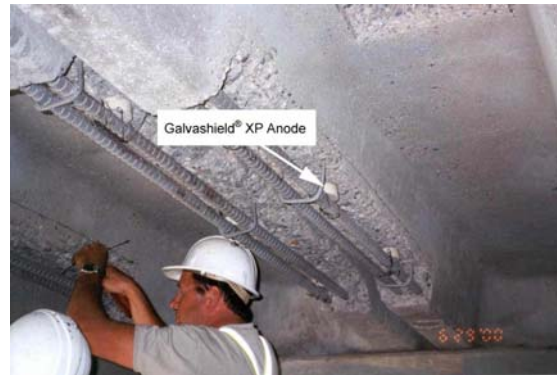
Concrete Girder Repair – Anodes tied to steel inside girder repair
