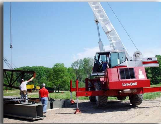
Joint training of iron workers and crane operators
