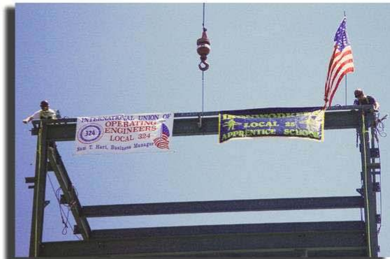
Topping out the training frame
