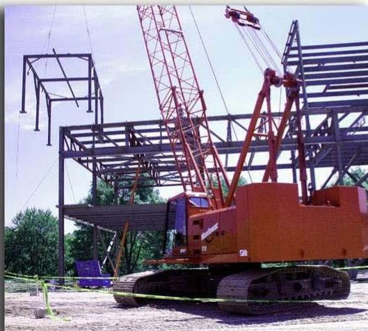
Old training frame (left) used as penthouse on new training frame
