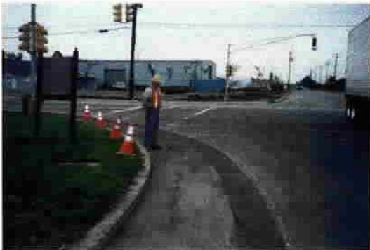
The Street Trencher can maneuver around obstacles and the grindings can be compacted to drive on.
