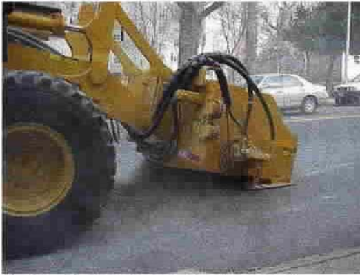
The Street Trencher saw cuts and grinds in one pass.
