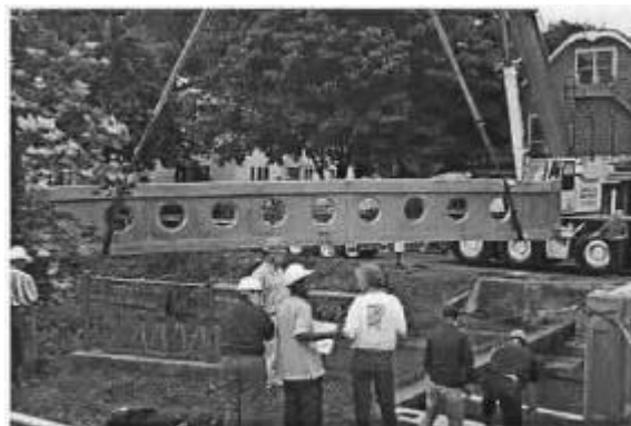
Installation of Carl Sagan Pedestrian Bridge in Ithaca, New York (June 2000)
