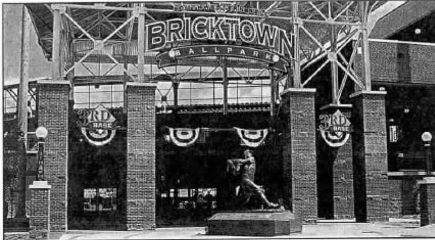
"We couldn't have done it without IMI," says Ken Lippert, whose firm, Continental Masonry, built Oklahoma City's new ballpark.
