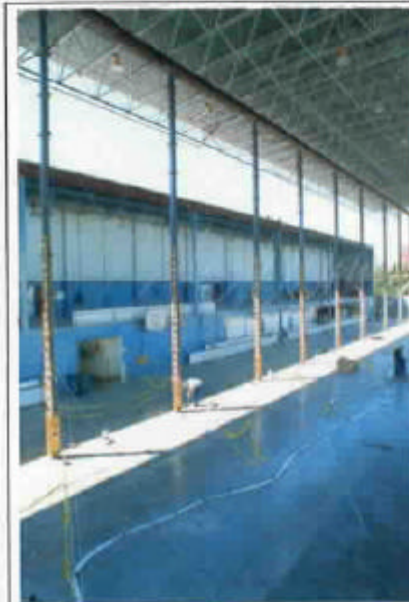
This portion of an existing mall in Spokane, WA was in need of a tenant until the owners of Future Shop decided to occupy the space. However, for the electronics retailer to make efficient use of the building they had to raise the existing roof. In order for Future Shop to implement its warehouse style of retail they needed an extra 10 feet of ceiling clearance.
