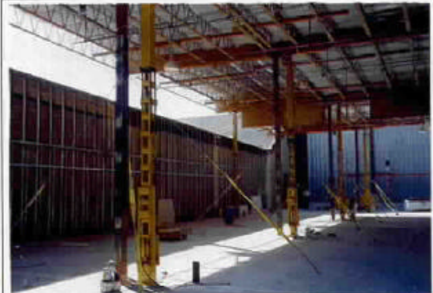
This portion of an existing mall in Spokane, WA was in need of a tenant until the owners of Future Shop decided to occupy the space. However, for the electronics retailer to make efficient use of the building they had to raise the existing roof. In order for Future Shop to implement its warehouse style of retail they needed an extra 10 feet of ceiling clearance.
