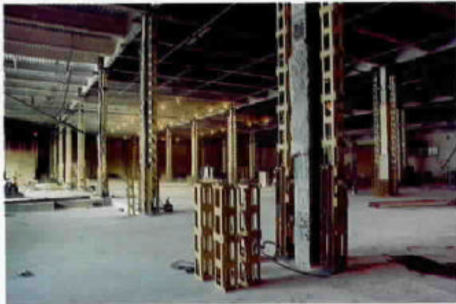
Wachovia Corporation, 16th largest bank in the country, purchased an abandoned tobacco processing plant near downtown Winston-Salem, NC from R.J. Reynolds with the intent to convert the building into an 800-employee office. The 50-foot tall building, built in 1982, had a 37,000 SF floor at mid-level. We converted the two-story building into three stories by raising the existing floor and building an additional one below it.
