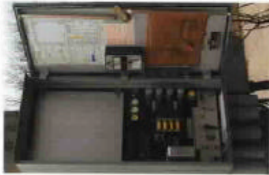
Base of Pole
