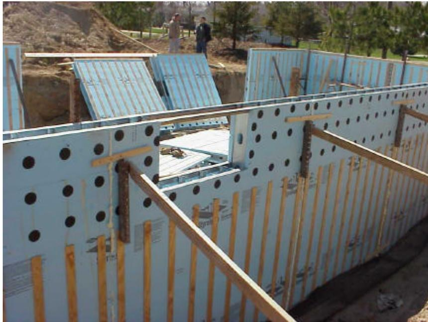
Steel studs provide vertical steel reinforcement to the concrete mass and reduce flexural cracking caused by lateral pressure. Knockouts in the stud allow concrete to flow horizontally, and accommodate placement of horizontal re-rod at 24" centers, reducing the incidence of shrinkage cracks.
