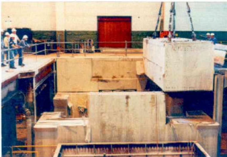
Figure 3 (left). Lifting of last segment, piece #1 on figure 1 (130 tons). Note clean surfaces on top of remaining piers, facilitating new construction.
