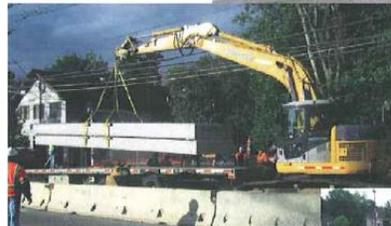
The 2,000 lbs beams are off-loaded two at a time and then set in place using a small excavator. All six beams were set in less than 4 hours.
