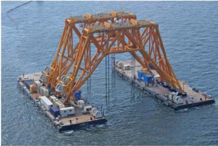
VERSABAR 4,000 Ton DECK SALVAGE SYSTEM "BOTTOM FEEDER" Gulf of Mexico, 2007
