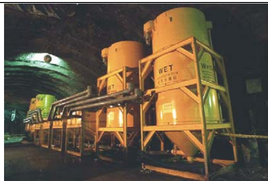
WetSep installed in Taiwan Pinglin Tunnel Project 250M underground
