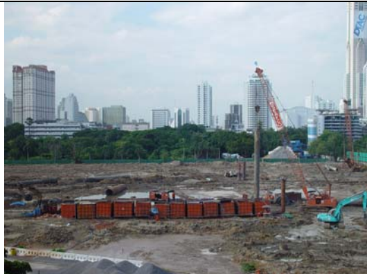
Foundation Project in Bangkok used numbers of sedimentation tank
