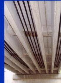
In addition to internal prestressing, each Structure B beam was externally post-tensioned with (4)-40mm (1.6 in.) diameter CFRP cables.
