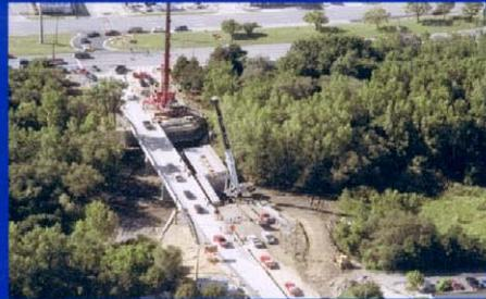
Two 500-ton mobile cranes were used to set the double-tee beams for Structure B.
