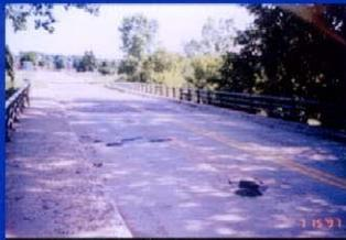
July 1997 - Existing bridge road surface shows significant deterioration.
