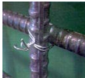
Figure 4. Photo of tied joint.
