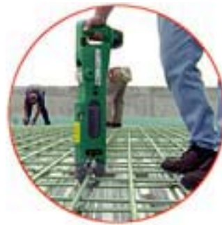
Figure 2. Demo of U-Tier being used.
