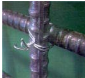
Figure 4. Photo of tied joint.
