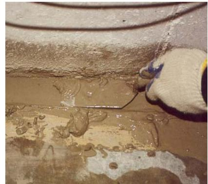
Installing positive electrode (anode) in groove at wall/floor junction of concrete
