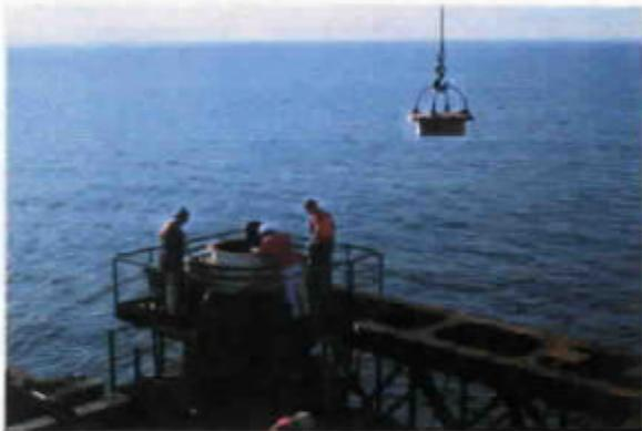
3. When the caisson was dry, a smaller pipe was inserted into the caisson and a diver was lifted by mancatcher into the pipe. When he reached the top of the diffuser, he opened the manhole cover that separated the diffuser from the outfall tunnel below. A crane lifted the cover away from the manhole.
