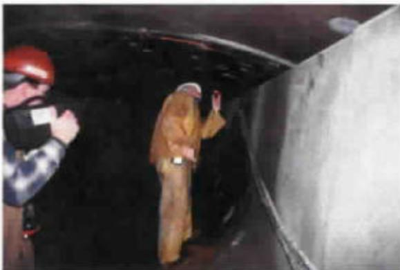
5. When the air was deemed sufficient for workers, a crew of divers went into the tunnel and within five days removed the remaining safety plugs that separated the tunnel from its 55-riser-pipe diffuser system.
