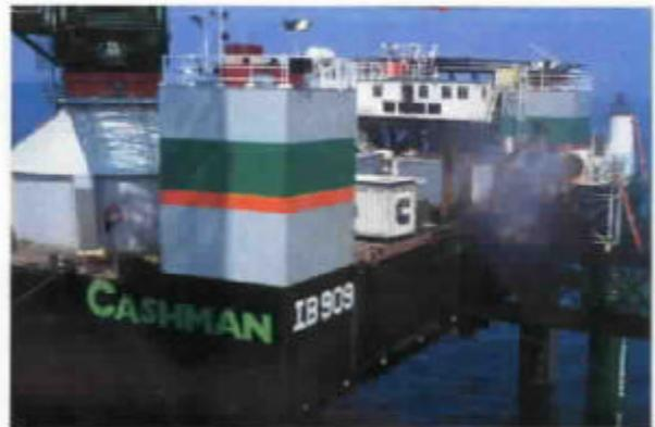
4. Once an opening was made into the tunnel, air was blown in from the Deer Island shaft and exhausted out through the newly-installed pipe at the diffuser.
