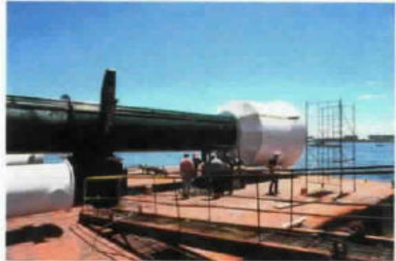
2. The caisson was 140-foot-long and 48-inches in diameter. The end of the caisson featured a bell-shaped construction that rested over a diffuser cap on the seafloor. An inflated rubber seal around the bottom prevented leakage. When the caisson was in place, all the water was pumped out of it.
