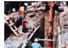
Forward movement is enabled by relaxing the spanning struts separating the front sidewalls, while maintaining pressure in the rear section. With the rear sidewalls serving as a thrust pad, the travel jacks are extended, pushing the front sidewalls ahead up to 8 inches. The front spanning struts are then extended to anchor the front section, the rear struts are relaxed, and the travel jacks pull the rear section into place with the front section.
