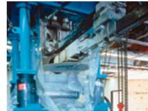
The system was devised to carry column loads while concrete segments were removed and isolators inserted, was developed by engineers at Adams & Smith. Friction yokes gripped each column, above and below the segment to be removed. Four 500-ton hydraulic jacks carried the column load, enabling full column support without bulky shoring.
